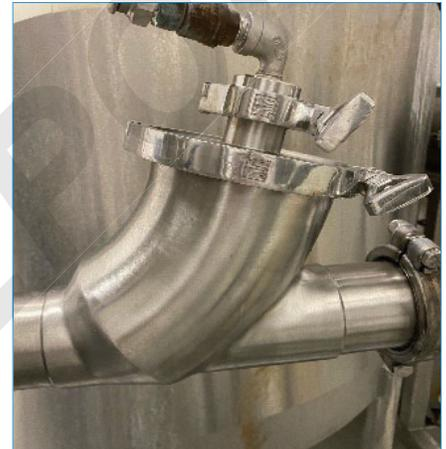
Figure 3. Ball Check Valve 1
