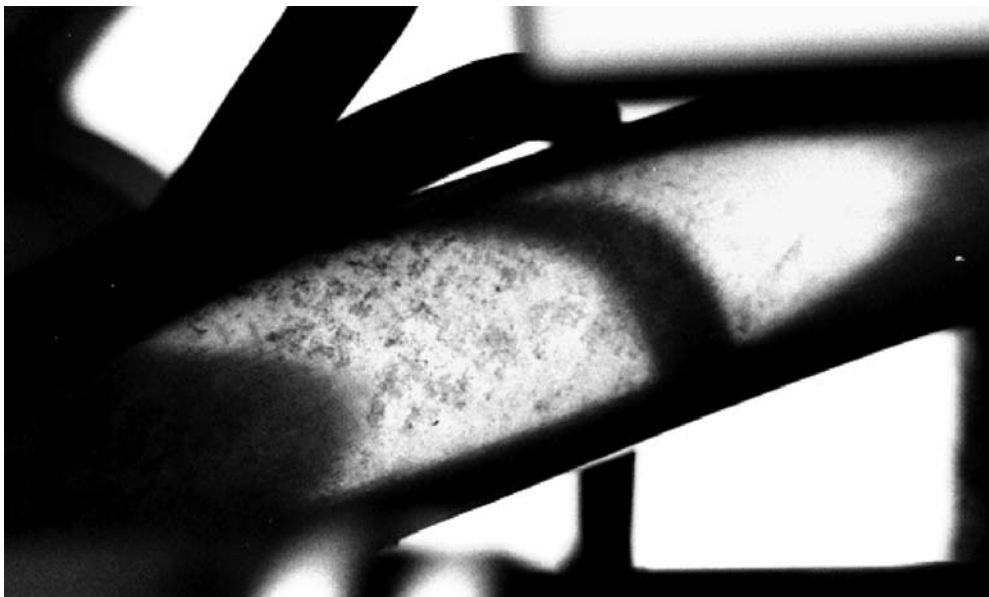
Figure 8.1 Visible biofilm on internal pipework of a hot tub, two weeks after installation
